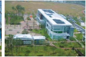
Yongin-Youngduk sewage treatment plant (13,000 tons per day)
