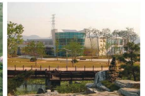
Kimpo-Yangchon industrial complex wastewater treatment plant (3,400 tons per day)
