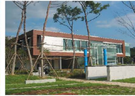
Siheung-Neunggok sewage treatment plant (7,000 tons per day)
